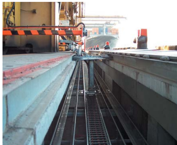
A large crane with up to 2,625 ft of travel
