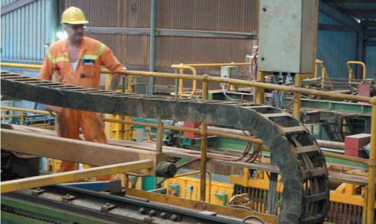
Three Energy Chains® in operation 24 hours a day for more than 4 years in a brick plant
