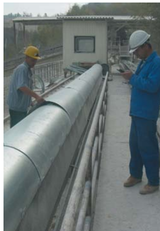
Steel construction for a spreader in a lime plant
