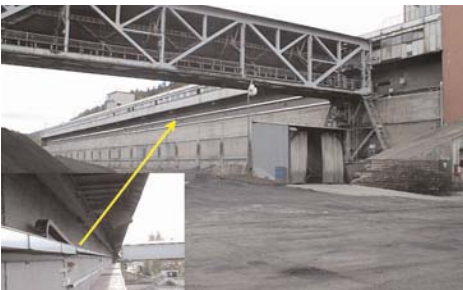
Power supply for transport of coal to a dump
