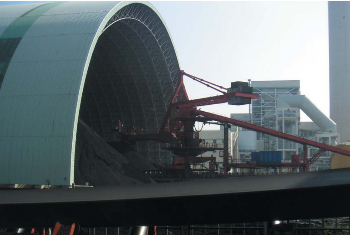
Supply of the bucket-wheel reclaimers using igus® Energy Chains®
